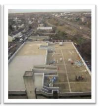
**The outcome:** The Apex Tower Car Park was successfully refurbished, and **APA** provided the Client with a high-quality anti-slip waterproof deck system (complete with a 10-year warranty), providing a sealed top deck and ensuring enhanced protection from water borne chlorides.
